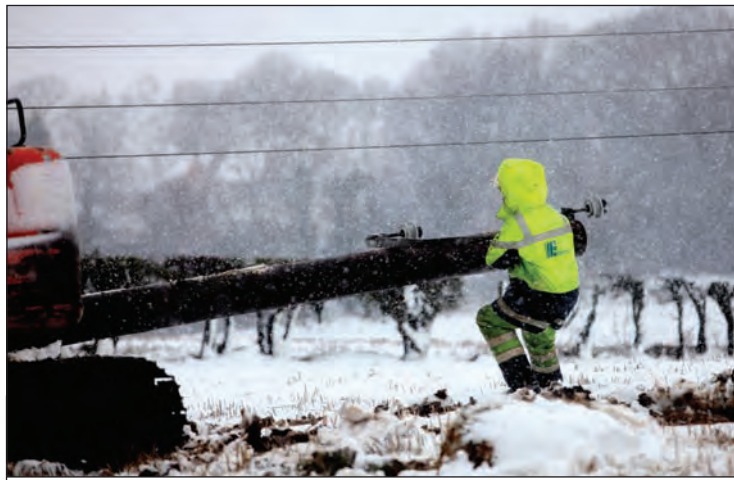
NIE crews out from first light restoring power supplies
